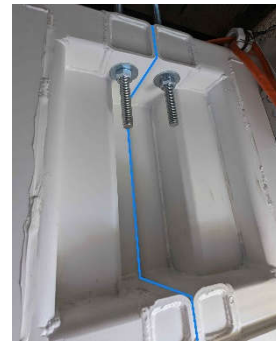
Caulk at exterior seams.
