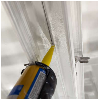
Caulk at ceiling grid seams.
